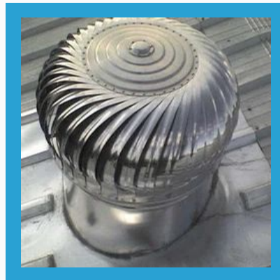
Roof Air Ventilator
