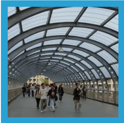
Polycarbonate Arch Roofing Work
