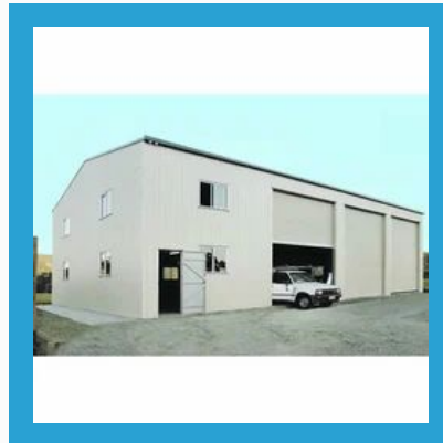
Prefabricated Steel Shed
