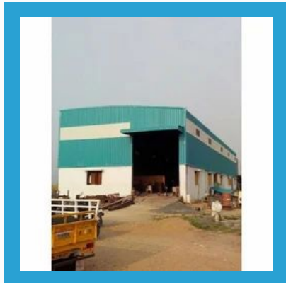
Prefabricated Factory Shed
